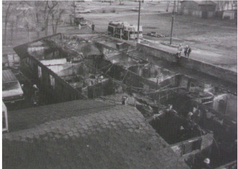
On March 4, 1991, ten elderly residents died in the Crystal Springs Nursing Home fire in Colorado Springs. Inadequate fire codes were found to be a contributing factor.
