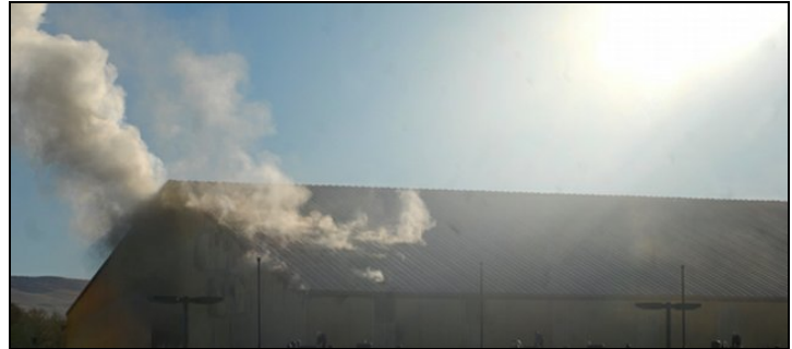
Smoke billowed out of the northeast side of the Road and Bridge Department's County Shop on Saturday afternoon. Photo by Jerry Raehal
