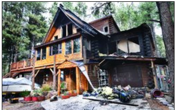
A Forest Lakes home north of Bayfield was partially destroyed during a fire Monday night. Jerry McBride, Durango Herald
